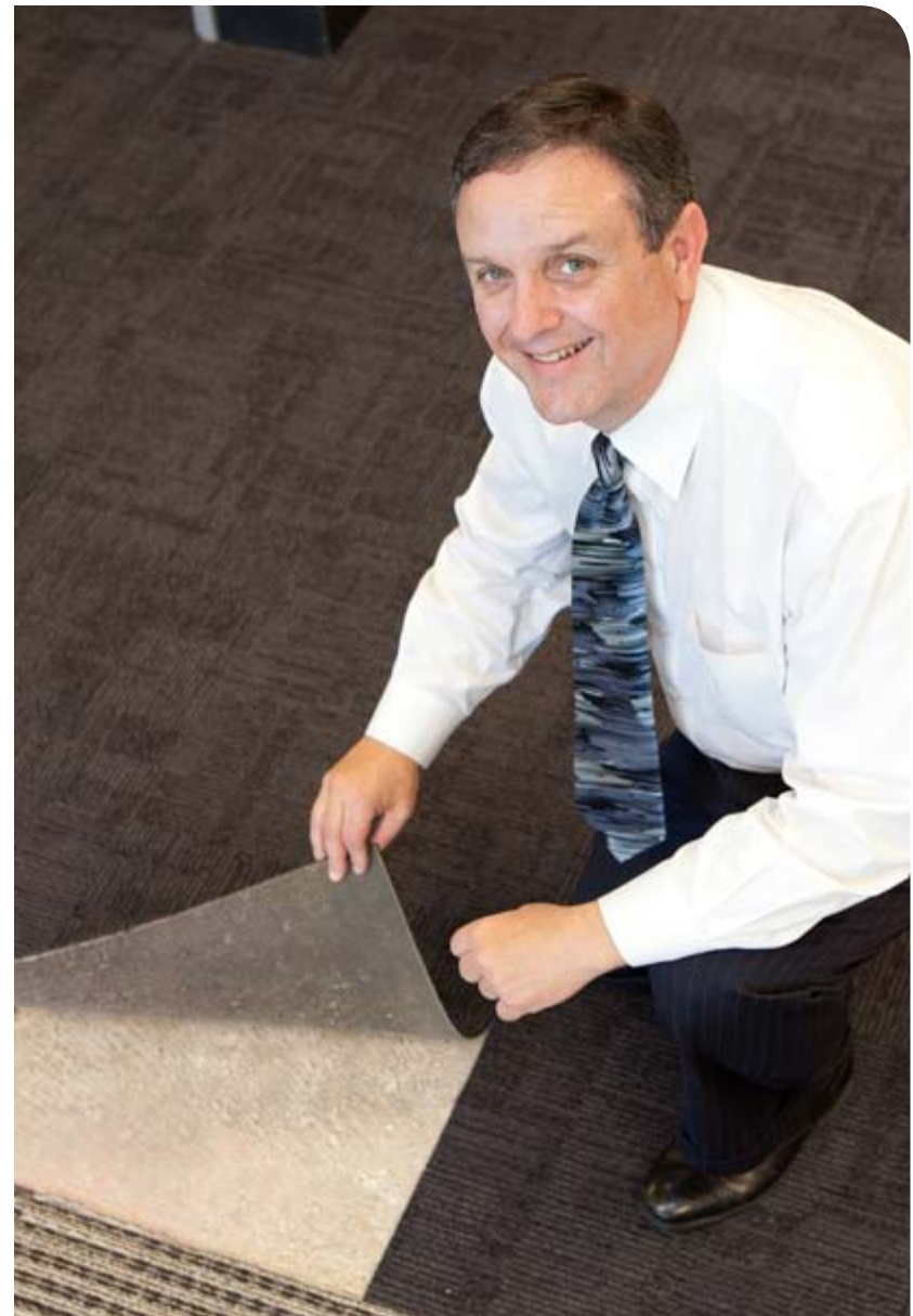
Regional project manager for Real Estate and Facilities Rob Boga demonstrates one of the benefits of Cool Carpet. Because it doesn't require glue, it exudes fewer chemical fumes than traditional carpet.
